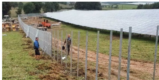
Erection of the complete fence system
